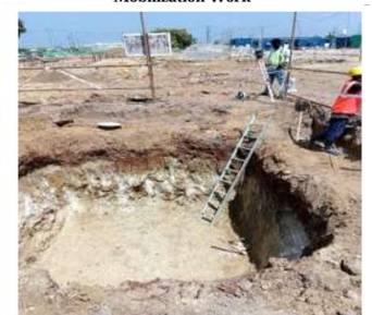
Footing Levelling and PCC Marking Work
