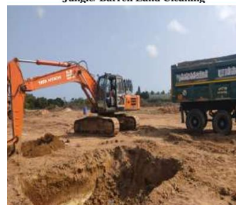
Earth work Excavation
