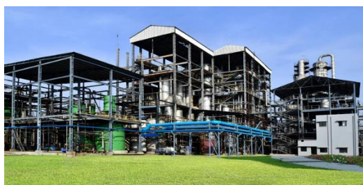
Sameerwadi Manufacturing Facility
