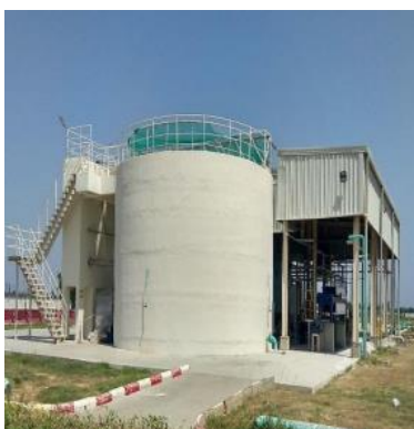
Pre-treatment clarification & pumping system
