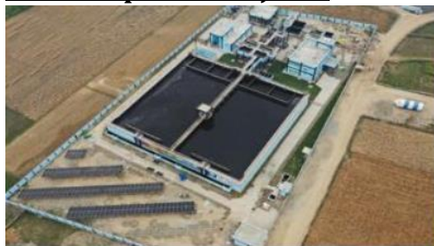
42+20+1 MLD Bareilly UP (includes solar plant)
