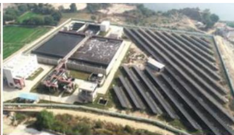
30 MLD STP Kota Rajasthan (includes solar plant)
