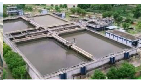
52 MLD STP at Bhatinda Punjab
