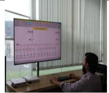
SCADA Monitoring of Distribution System
