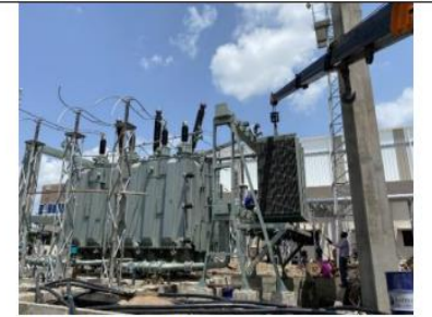
Installation Of Power Transformers
