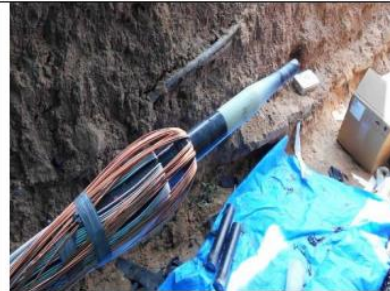
EHV/MV/HV/LV Cable Joining
