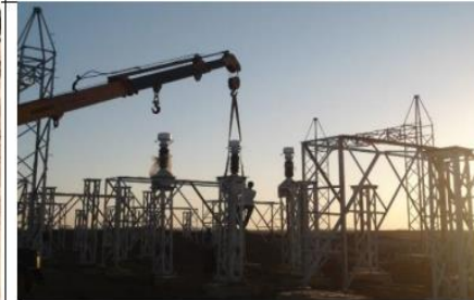
Switchyard Installation Work
