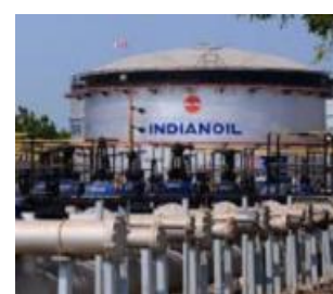
IOCL Project, Paradip
